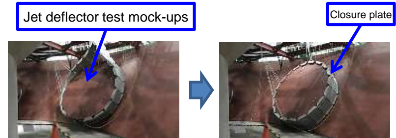
Preliminary test status of closure plate installation
